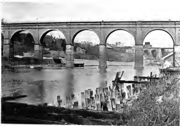
A CLOSE UP SHOWING THE RIVER PIERS WHICH THE WAR DEPARTMENT CLAIMS FORM AN UNREASONABLE OBSTRUCTION TO NAVIGATION.
